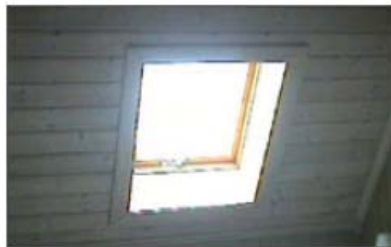
Image shows air leaks between the ceiling and the window.
